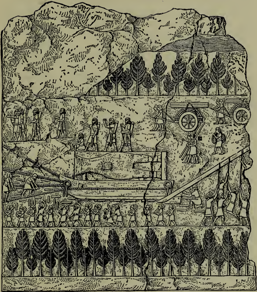
64.—HALF-SCULPTURED WINGED BULL DRAGGED ALONG ON A SLEDGE ON GREASED WOODEN ROLLS. OVERSEERS DRIVING CAPTIVES TO WORK.
